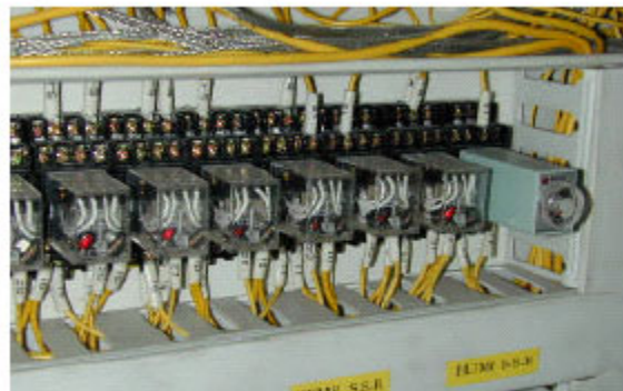
Figure 15: LED Relays
